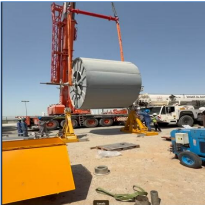
Load assessment to confirm safe lifting capacity
